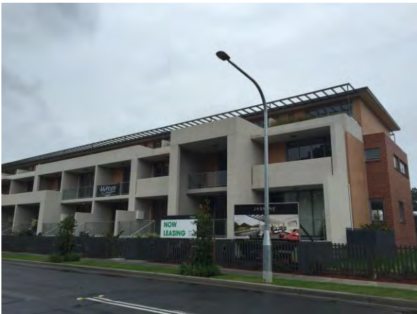
PICTURE 2.7 – NEW APARTMENTS, JASMINE STREET
