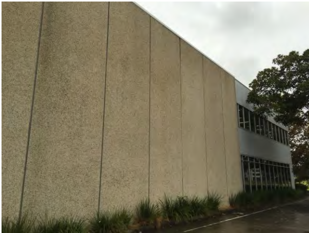
PICTURE 2.3 – TYPICAL BUILDING CONSTRUCTION
